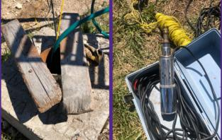
KCARE Watershed specialists, in partnership with John Redmond WRAPS and a local landowner work to install a pump in an existing well and two solar panels, mounted on a windmill tower. This system provides reliable water for livestock in this pasture.
