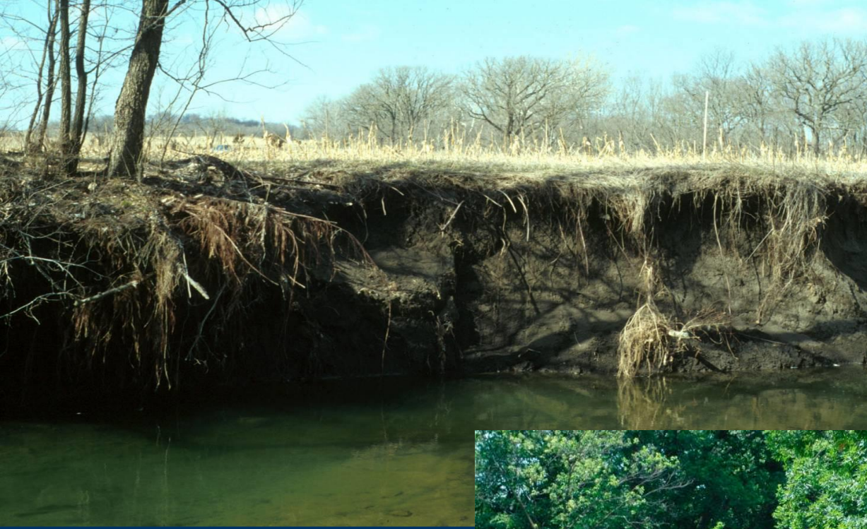
Crow Creek February 1999, before cedar revetment was installed.
