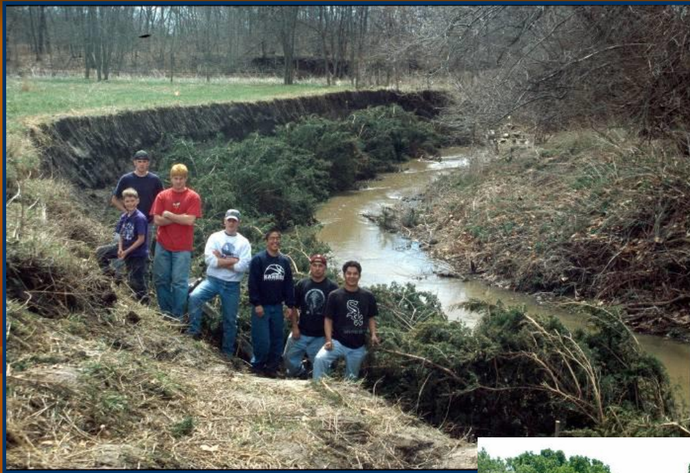
Little Soldier Creek, March 2000, immediately after cedar revetment was installed.
