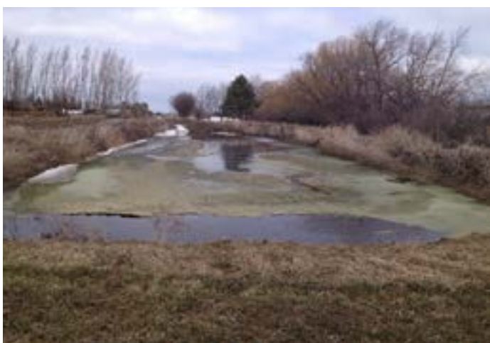
Figure 2. An effluent containment pond. Ponds are designed to hold water for a period of 270 days plus a 24-hour, 25-year rain event, while allowing at least an additional foot of freeboard.
