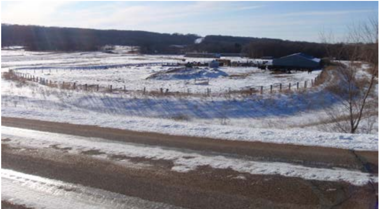
Figure 7. A clean-water diversion constructed at the base of a hill. The diversion prevents contamination of clean upslope runoff with manure in the feeding area.
